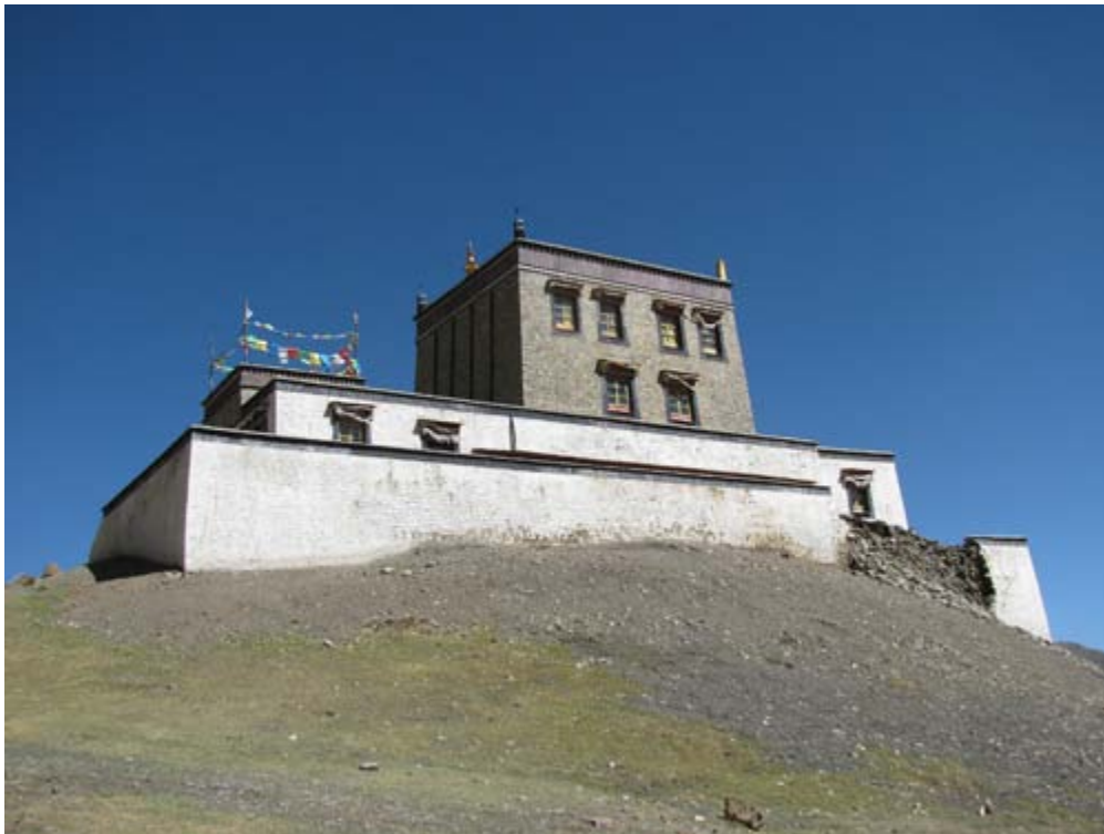
Gyangdrak monastery. Note the crumbling apron-wall on the right side of the structure.
